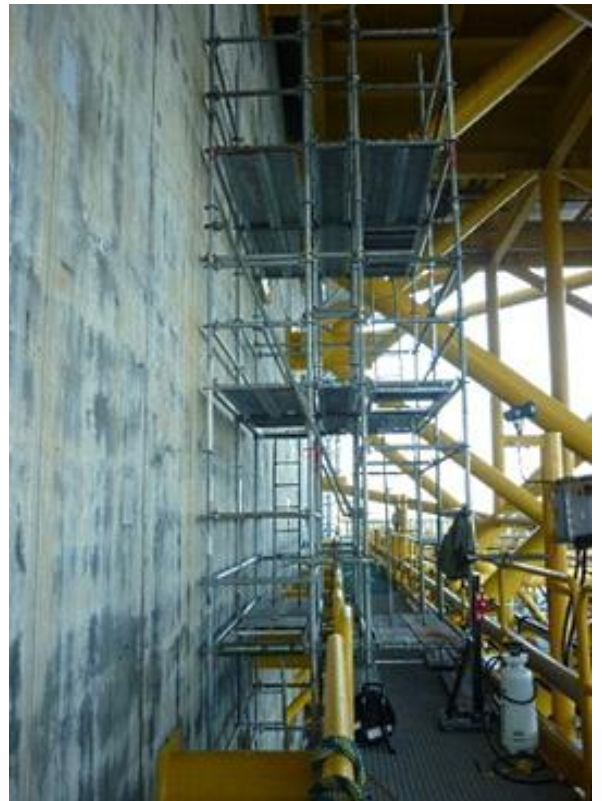
Fig. 7 - Activities on concrete walls of a Gravity Based Structure
