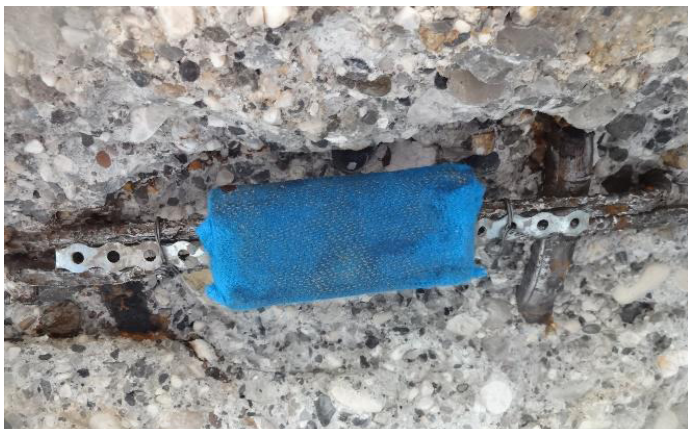
Zinc galvanic anodes for rebar cathodic protection
