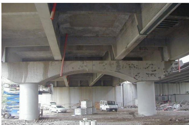
Bridge architraves protected by an ICCP system
