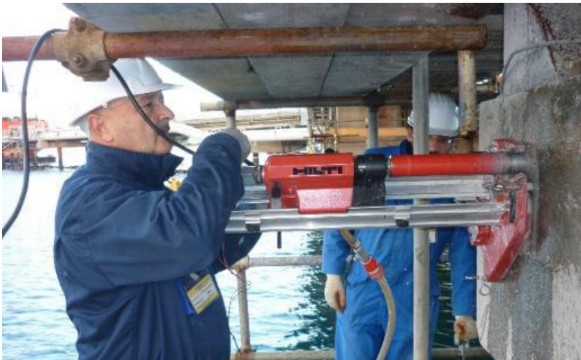
Core drilling
