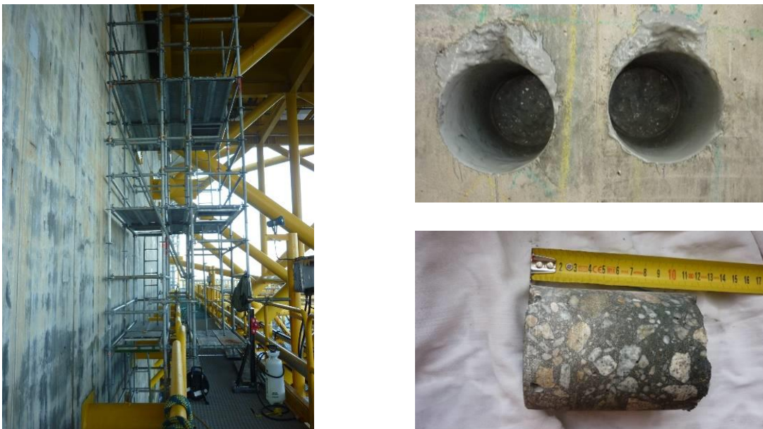
Figure 3: Concrete coring campaign.
