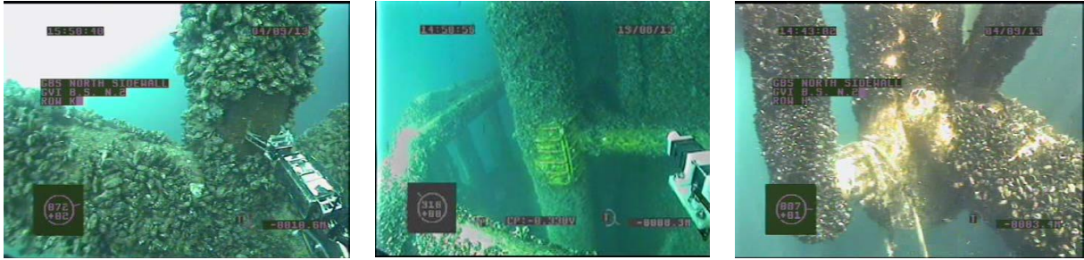
Figure 5: Underwater close visual inspection of mechanical outfitting.
